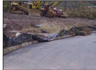
**Exposed stock piles and soil** can easily run off construction sites resulting in costly repairs clogging drainage structures.
