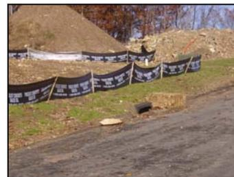
A simple **tarp** over this stock pile and **geotextiles** can help to avoid this problem.
