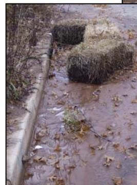
**Straw bales** can easily shift during storm events allowing sediment to enter nearby stormdrains.
