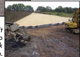
Geotextile/silt fence used to stabilize bank erosion.
